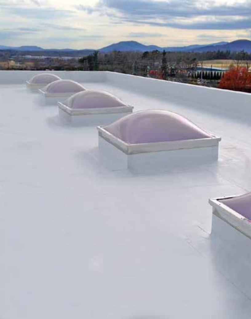
Apple Tree Honda Fletcher, NC EcoSky Deck Mount Units, 60" x 60", 18" Curbs. Glazing: Satin Sky® over Clear Acrylic. Finish: Mill.
