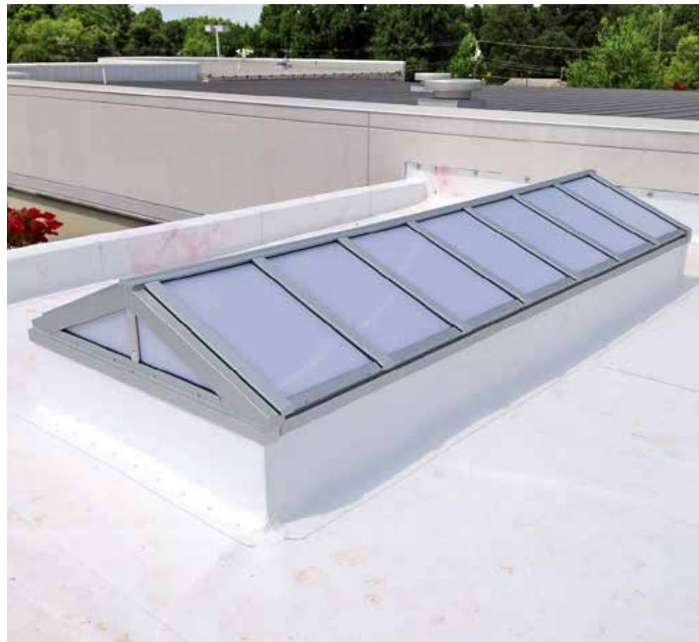
Rice Toyota Greensboro, NC Horizon S-Series, Classic Framing System, Double Pitch, 13' x 5', 5:12 Pitch. Glazing: 25mm Opal Multiwall Polycarbonate. Finish: Clear Anodized.
