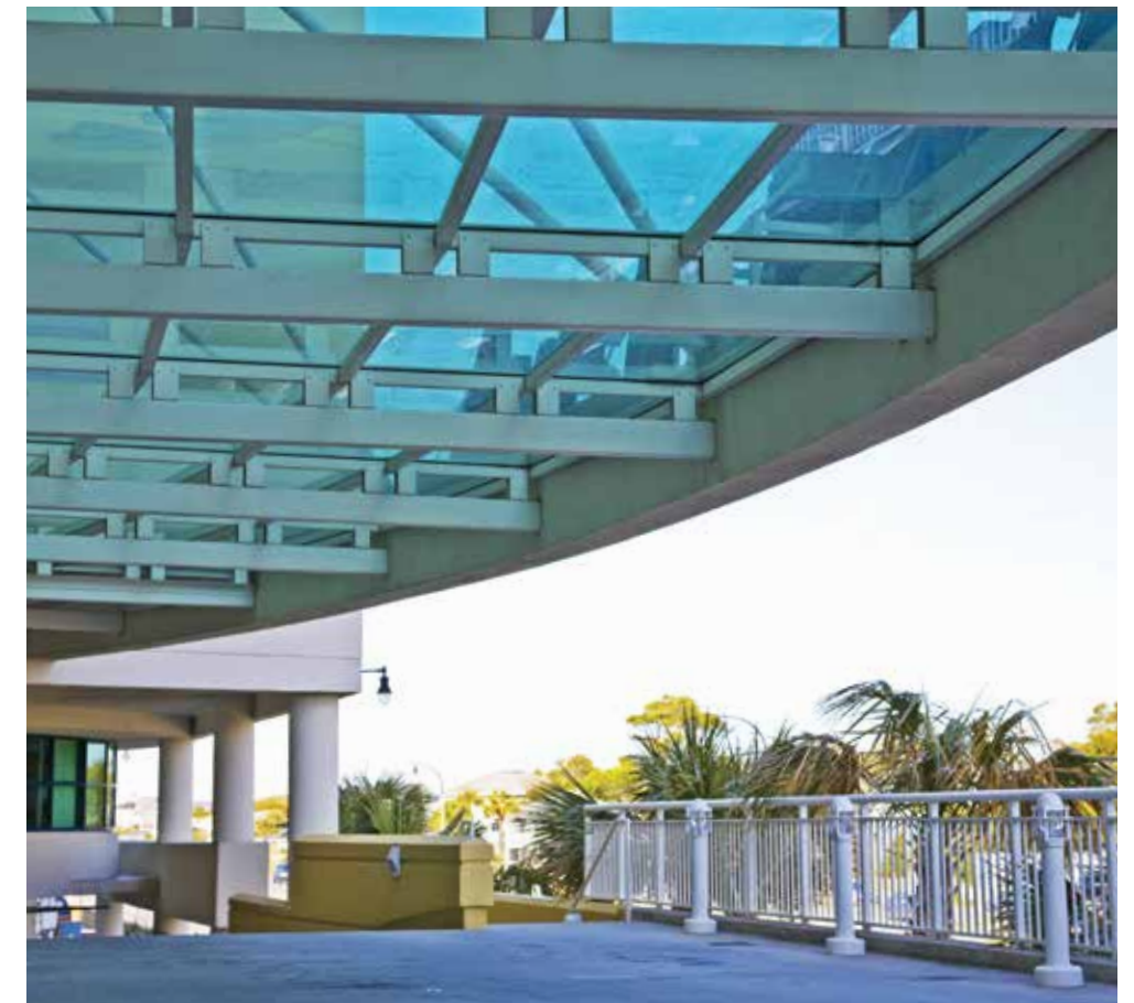
Avista Resort North Myrtle Beach, SC Glass Canopy, Pinnacle 350 Single Pitch, 13'9" x 60'. Finish: Kynar Bone White.
