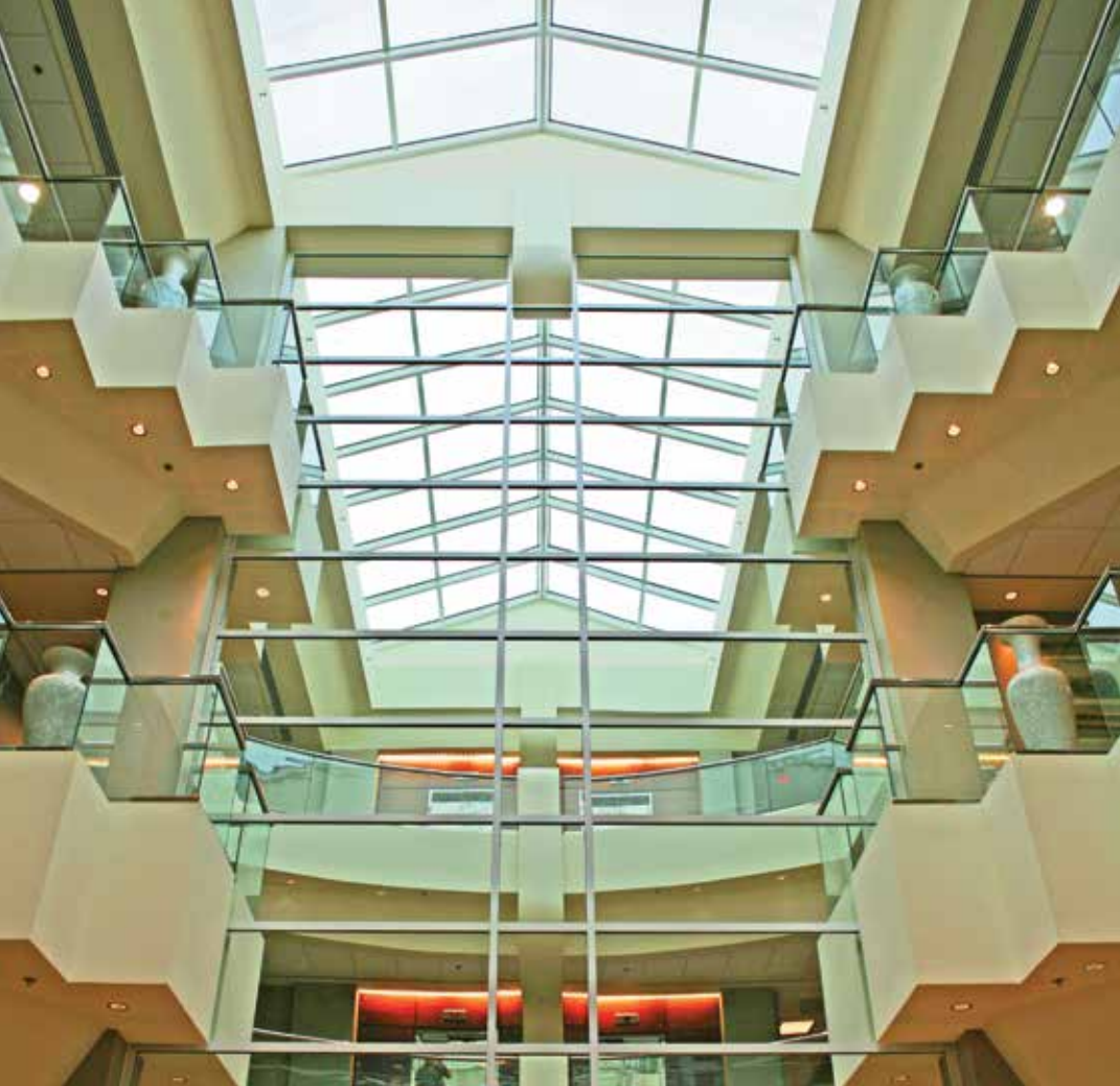
600 Concourse Jackson, MS Barlow Eddy Jenkins Pinnacle 600 Double Pitch, 23' x 33'. Finish: Kynar 500 Bone White.
