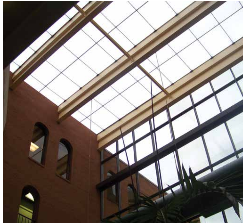
Iona Kent County Courthouse Grand Rapids, MI Barrel Vault with Vertical Ends, (5) 9' x 36'. Glazing: Clear Acrylic over 25mm Clear Polycarbonate Panels Filled with Lumira Aerogel. Finish: Dark Bronze Anodize.
