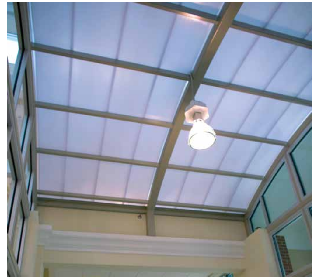
Ingles Store Chesney, SC Little & Associates Deck Mount Units, 60" x 60", 14" Curbs. Glazing: Pyramid Clear Acrylic over 16mm Multiwall Polycarbonate Panels filled with Lumira® Aerogel. Finish: Mill. Horizon C-Series Low Rise Vault, 15' x 24'. Glazing: 20mm Opal Standing Seam Multiwall Polycarbonate.
