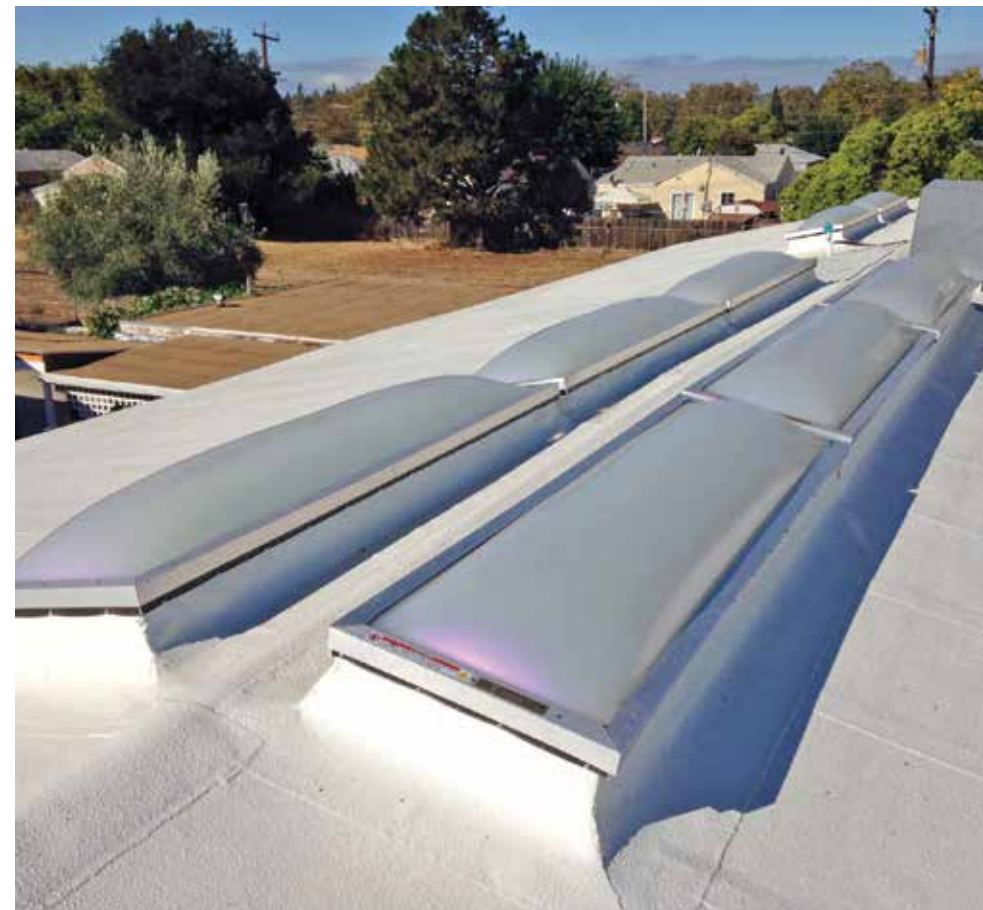
City of Vallejo Library & Fire Station Vallejo, CA
