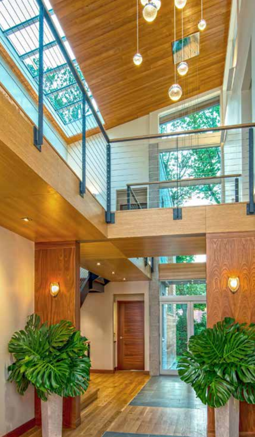
Englewood, NJ Robert Gross, AIA LEED | AP Low Profile Deck Mount (LPG), 14' x 4', 3:12 Pitch. Finish: Exterior Mill, Interior Baked Enamel Bone White.
