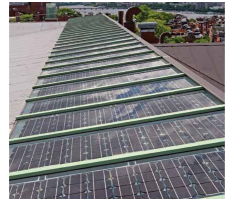
Traditional non-light transmitting photovoltaic glass was used in non-public areas.
