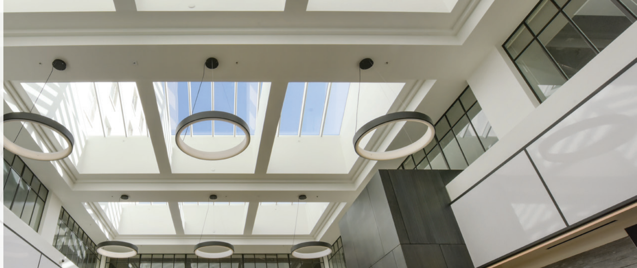
VMS Ridgelight, The Leamington Hotel, Oakland, CA
