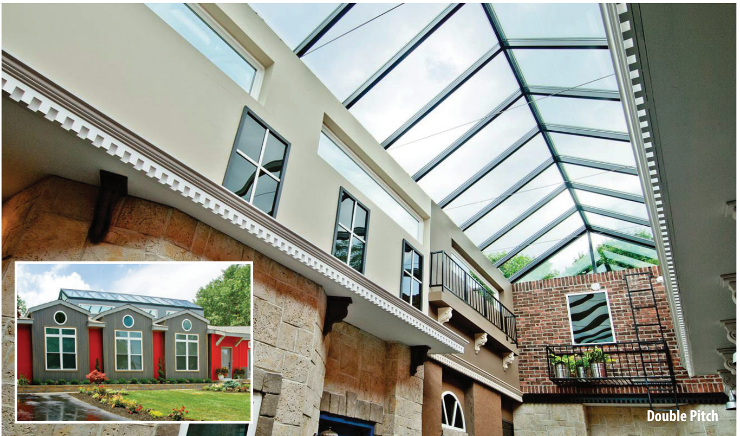
Extreme Makeover: Home Edition, East Setauket, NY Pinnacle 350 Framing System, Double Pitch, 12' x 36', 4:12 Pitch. Glazing: 1 \frac{1}{16} " IG. Finish: Kynar 500 Black.
