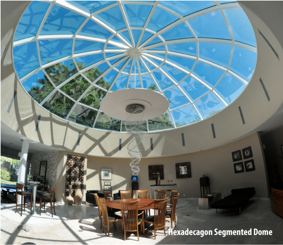
Left: Dallas, TX Pinnacle 600 Framing System, Segmented 16-Sided Polygon Dome, 30' 5" Diameter, 8' High. Glazing: 1 1/8" IG. Finish: Kynar 500 Quaker Bronze Exterior, Kynar 500 Bone White Interior. Right: Westerly, RI Classic Framing System, Custom 6' Hexagonal Pyramid, 7:12 Pitch. Glazing: 1 1/8" IG. Finish: Kynar 500 Colonial White.
