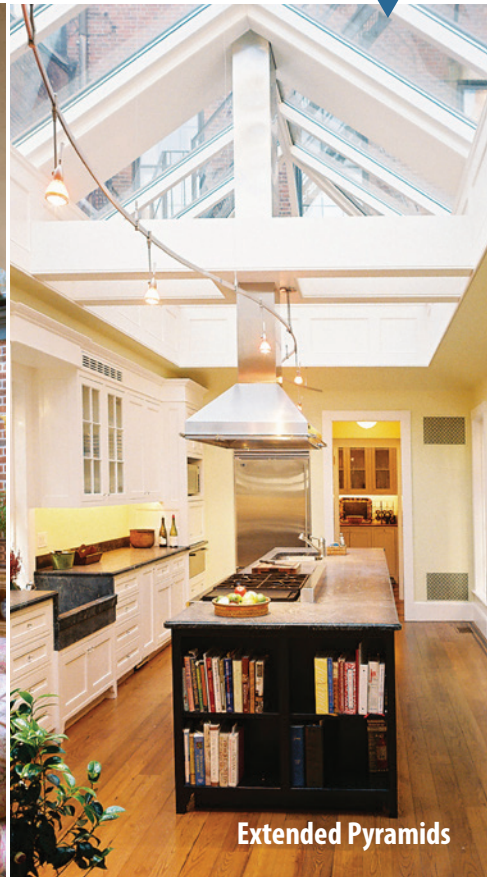
Left: Augusta, GA Hurricane Pinnacle 350 Framing System, Custom Half Extended Pyramid, 10' x 22', 4:12 Pitch. Glazing: 1½" IG Hurricane Rated. Finish: Kynar 500 Hartford Green Interior with Copper Cladding Exterior. Right: Boston, MA Pinnacle 350 Framing System, Extended Pyramid, 10' x 22', 4:12 Pitch. Glazing: 1½" IG. Finish: Kynar 500 Bone White Interior with Copper Cladding Exterior.
