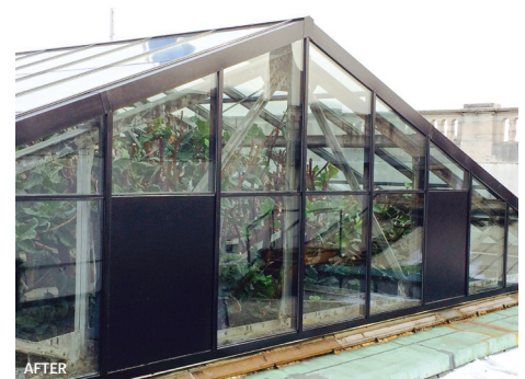
Before and after of the Atrium exterior.
