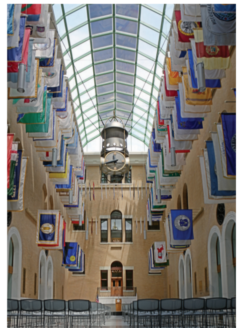
The large atrium skylight is a Pinnacle Segmented Vault with integrated photovoltaics in the center.
