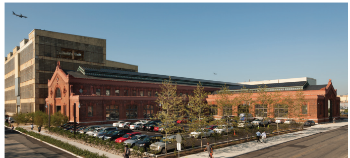
The dilapidated old building #18 was transformed into an inspiring, creative and light filled work space.
