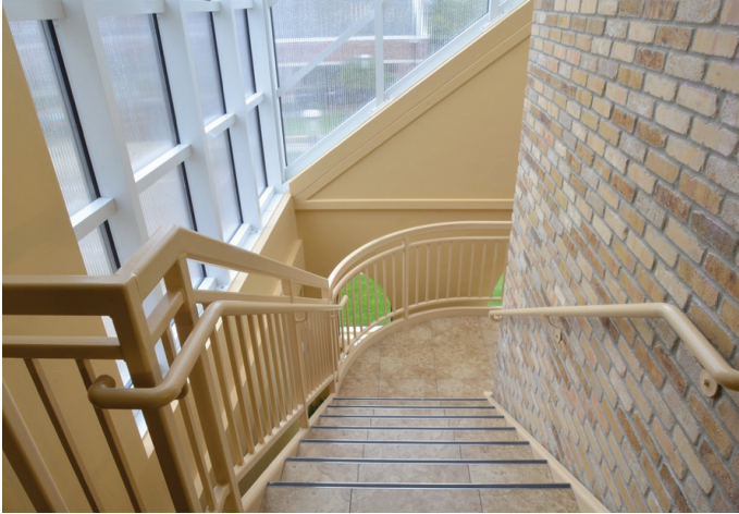
Atrium: Pinnacle 600 Double Pitch, 25mm Lexan™ Thermoclear™ Polycarbonate Panels (Filled with Lumira® Aerogel on Roof), Kynar Bone White Finish.
