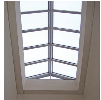
The larger skylight is a 12' 9" x 32' Pinnacle 350 double pitch with Horizon polycarbonate glazing at a 6:12 pitch. Two smaller skylights were 7' 6" x 13' 6" with a 6:12 pitch.
