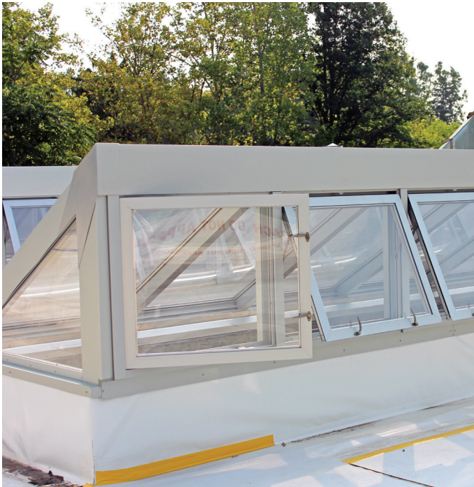
Awning type vents and casement windows enabled the food to be broadcast to the animals through the roof openings.
