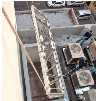
The larger skylight is a 12' 9" x 32' Pinnacle 350 double pitch with Horizon polycarbonate glazing at a 6:12 pitch. Two smaller skylights were 7' 6" x 13' 6" with a 6:12 pitch.
