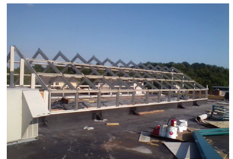
Wasco's Pinnacle unit skylight and SOLERA glazing combine for natural light and structural integrity in the Media Center.
