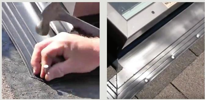
Snap the aluminum brackets (provided) in the groove found directly underneath the Ultraseal Flashing, spacing approximately 6" from corners (4" on 14" side) and in the middle of the side when 3 are used. Screw to deck with screws provided.
