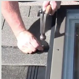
At the top: Place shingles OVER the flexible flange and the L-gasket as follows: First, nail an inverted shingle(s) across the width of the skylight (similar to use of starter shingle at roof edges). An inverted shingle would have bottom edge of shingle facing up the slope.
